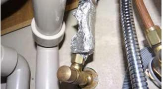
These two pictures show how the MiniTuner and the water pipe are isolated with the aluminium foil to avoid interferences.
